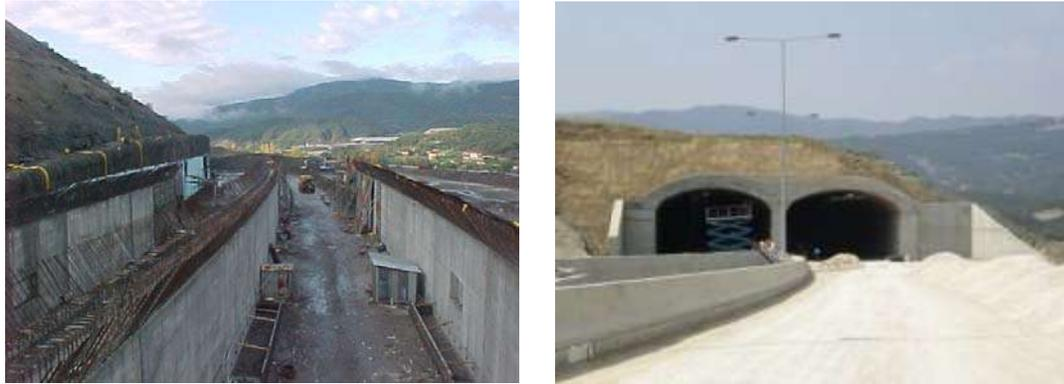
**Figure 8:** “Cut and Cover” tunnel
