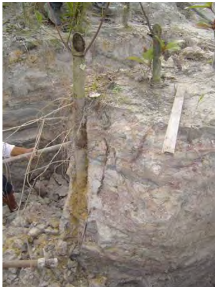
(a) An Ht pole during excavation
