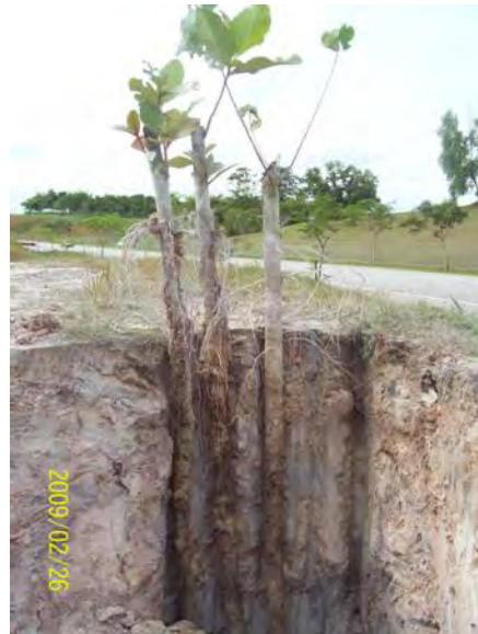
(b) Live poles after removing
