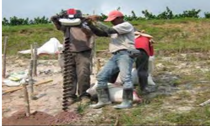
Figure 13: A two-man powered auger team preparing the pre-formed hole
