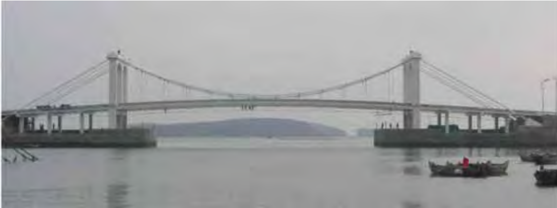
Figure 1: Xiaoping Island Bridge
