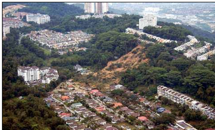
Figure 8: The 6 th December 2008 Bukit Antarabangsa, Ulu Klang, Malaysia landslide.
