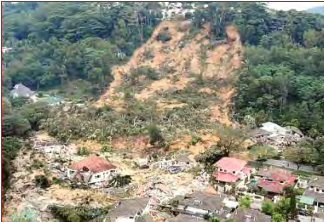
Figure 1: Overall View of the Bukit Antarabangsa Landslide
