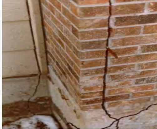
**Figure 5:** Cracks in exterior walls, as a result of upward soil expansion (<http://www.surevoid.com/...>, 2006).
