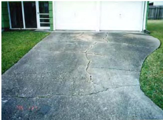
**Figure 3:** Residential driveway damaged by expansive soil (<http://www.surevoid.com/...>, 2006).
