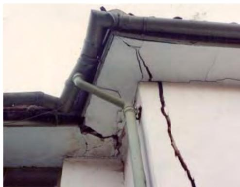
**Figure 4:** Structural damage to house caused by 'end lift' (Jones, 2011).
