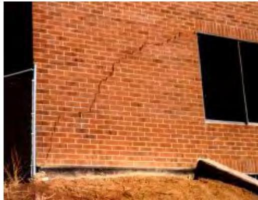
**Figure 6:** Major cracks in exterior walls at doors and windows (<http://www.surevoid.com/...>, 2006).
