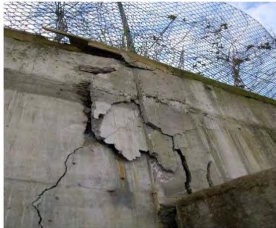
**Figure 18:** Collapse of the retaining wall
