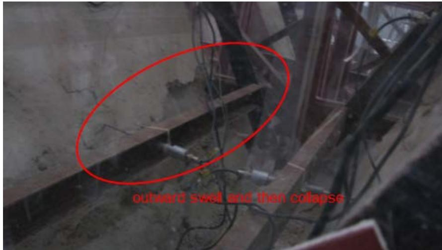
**Figure 4:** Bend and collapse in slope toe
