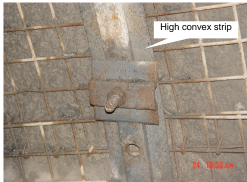
Figure 11: Field usages of the high convex strip in Hebi coal mine.
