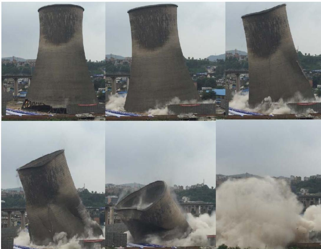
**Figure 8:** The videoed process of cooling tower collapse
