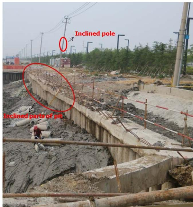
**Figure 2:** Scene photo of pit with large deformation
