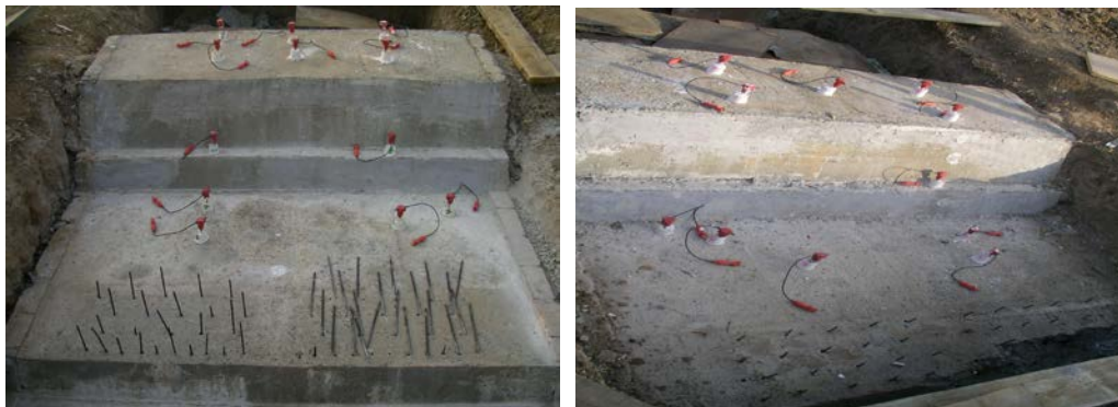
Figure 2: Concrete model and sensor installation
